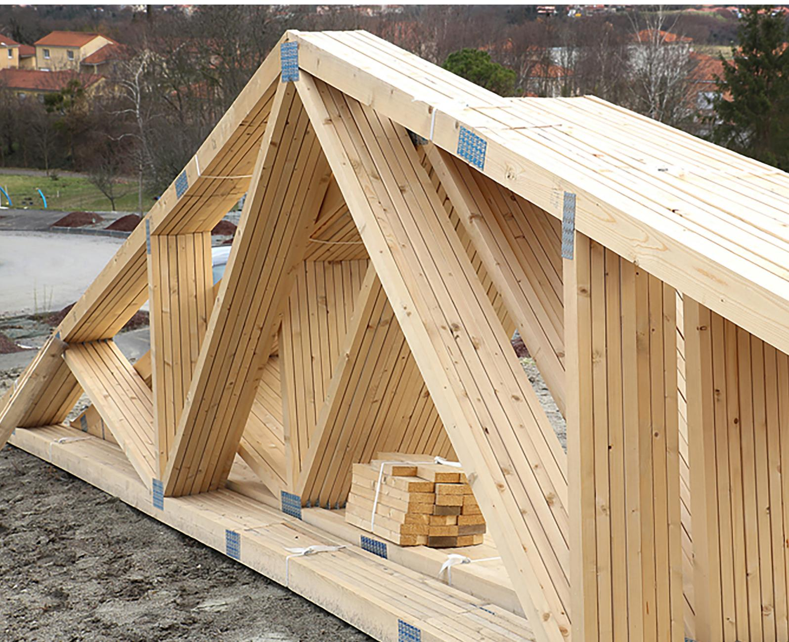
Metal connectors for timber structures
